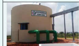
Pump House at Kanigiri Reservoir
